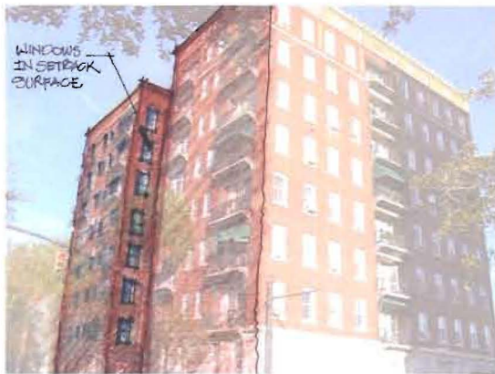
Setbacks in the mass of a large-scale building should introduce windows in the perpendicular surface.
