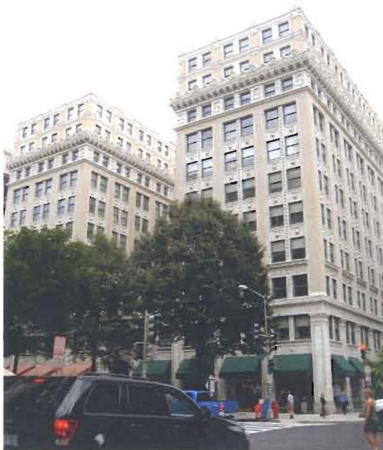
This building's mass is set back above the base level allowing light to penetrate interior spaces and providing relief in the streetwall.
