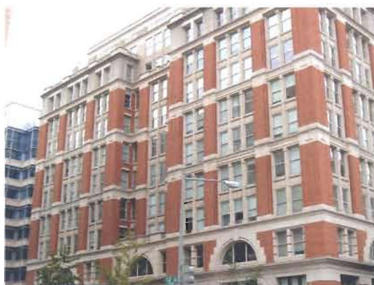
Combination of setbacks and materials are employed to create interest and variety in a large building.
