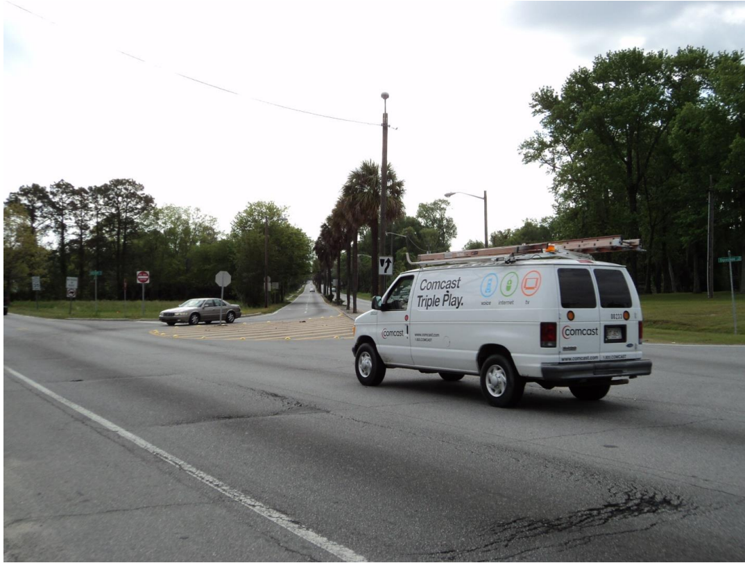
Figure 35 Segment 6 pavement conditions
