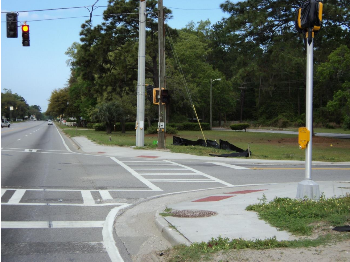
Figure 27 Crosswalk and Curb-cuts, Segment 3
