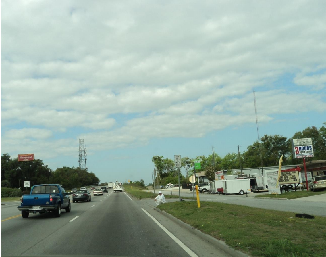
Figure 33 Frontage Road and Bus Stop Location, Segment 5
