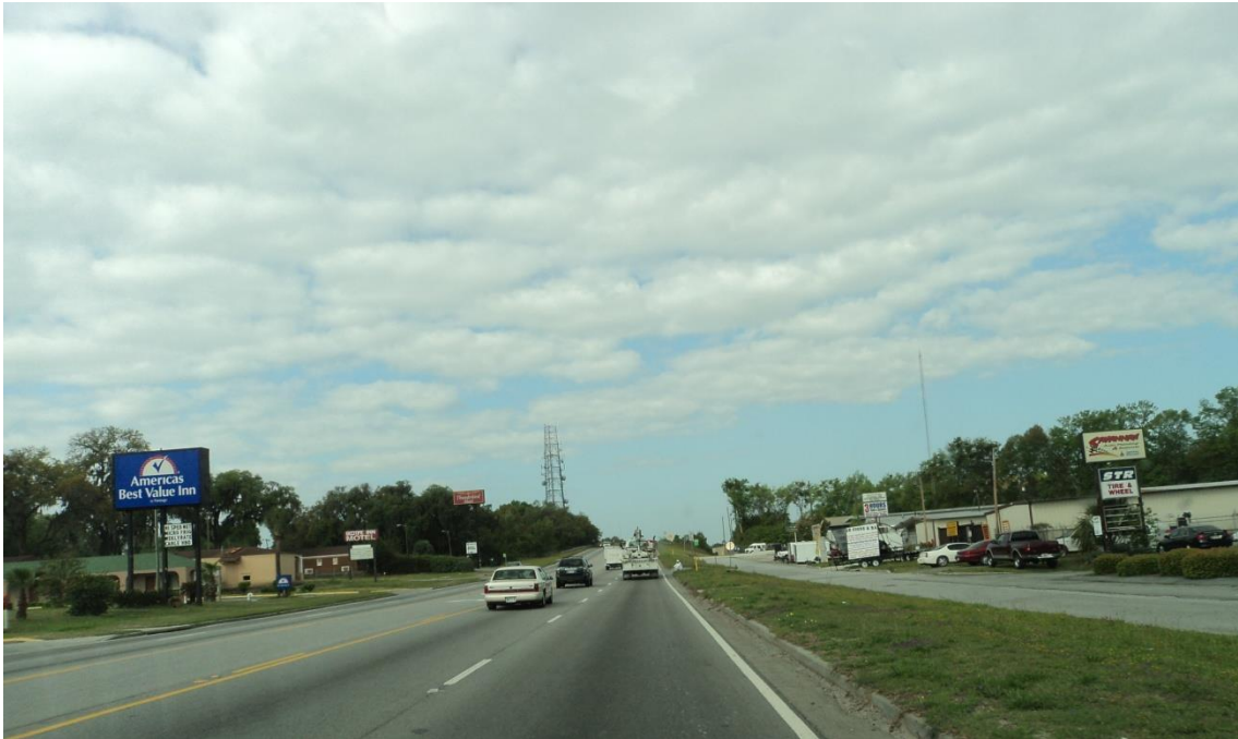
Figure 32 Frontage Road and Bus Stop Location, Segment 5
