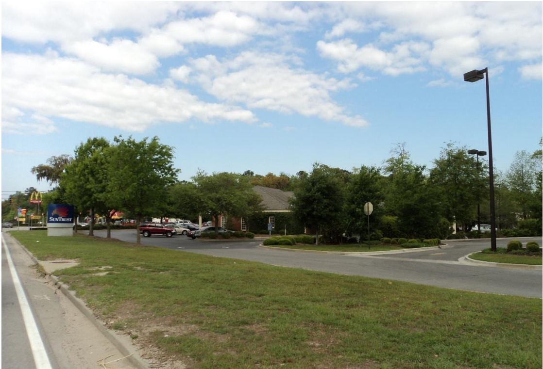
Figure 30 Recently Developed Commercial Area at Chatham Parkway with Frontage Road and Interparcel Access, Segment 4
