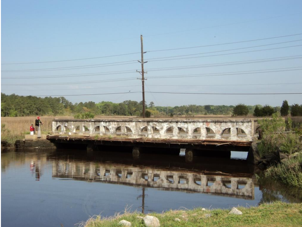
Figure 25 Segment 2 Salt Creek Boat Ramp and Park, Segment 2
