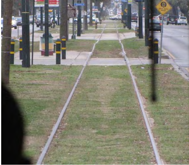
Figure 9. Off Street Operation; New Orleans, Louisiana
