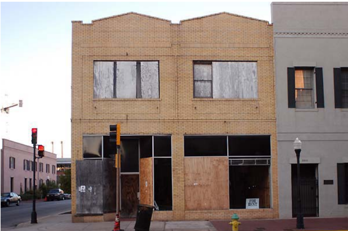
Front façade of building on West Broughton Street –Primary Façade
