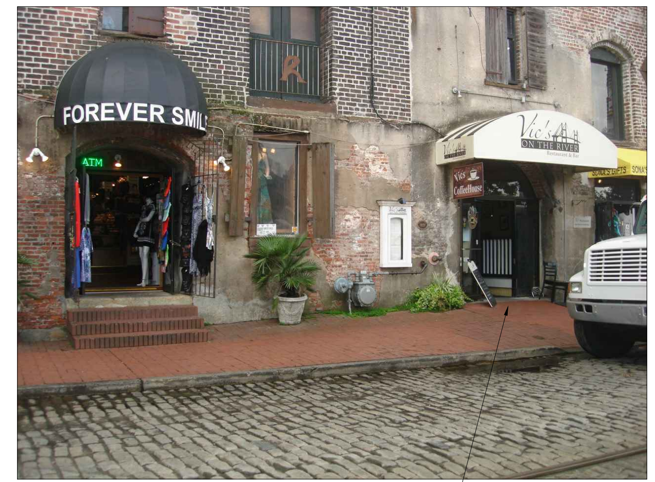
ADJACENT WEST PROPERTY SLOPED GRADE-LEVEL ENTRY AT EXISTING NEARBY ENTRANCE
