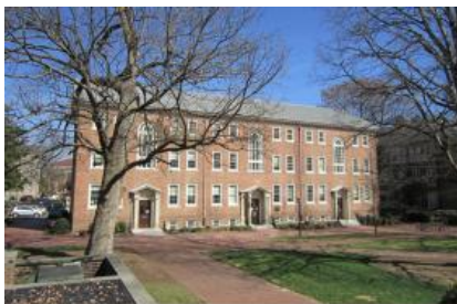
UNC Chapel Hill - Steele Building
