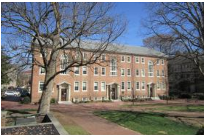
UNC Chapel Hill - Steele Building
