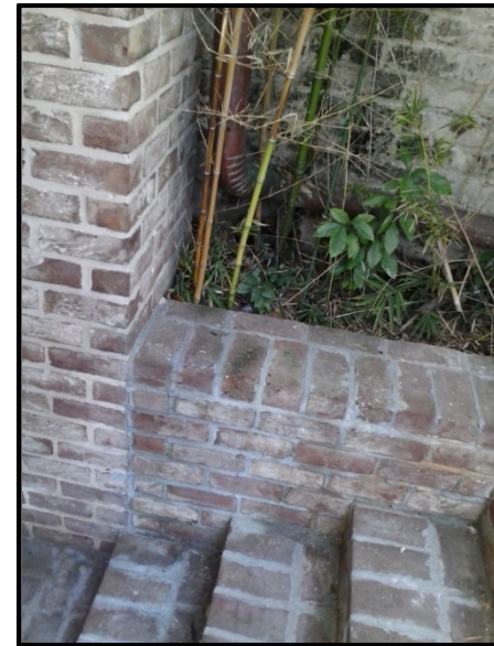
Example of steps leading down to gate
