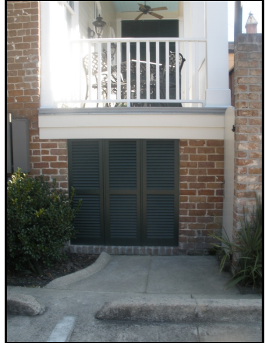
Example of louver panels for east door
