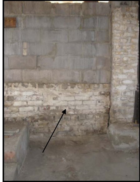
Interior where the iron gate will be
