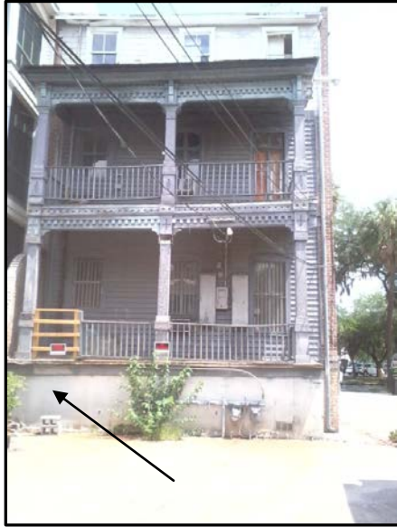
Exterior view where the iron gate will be
