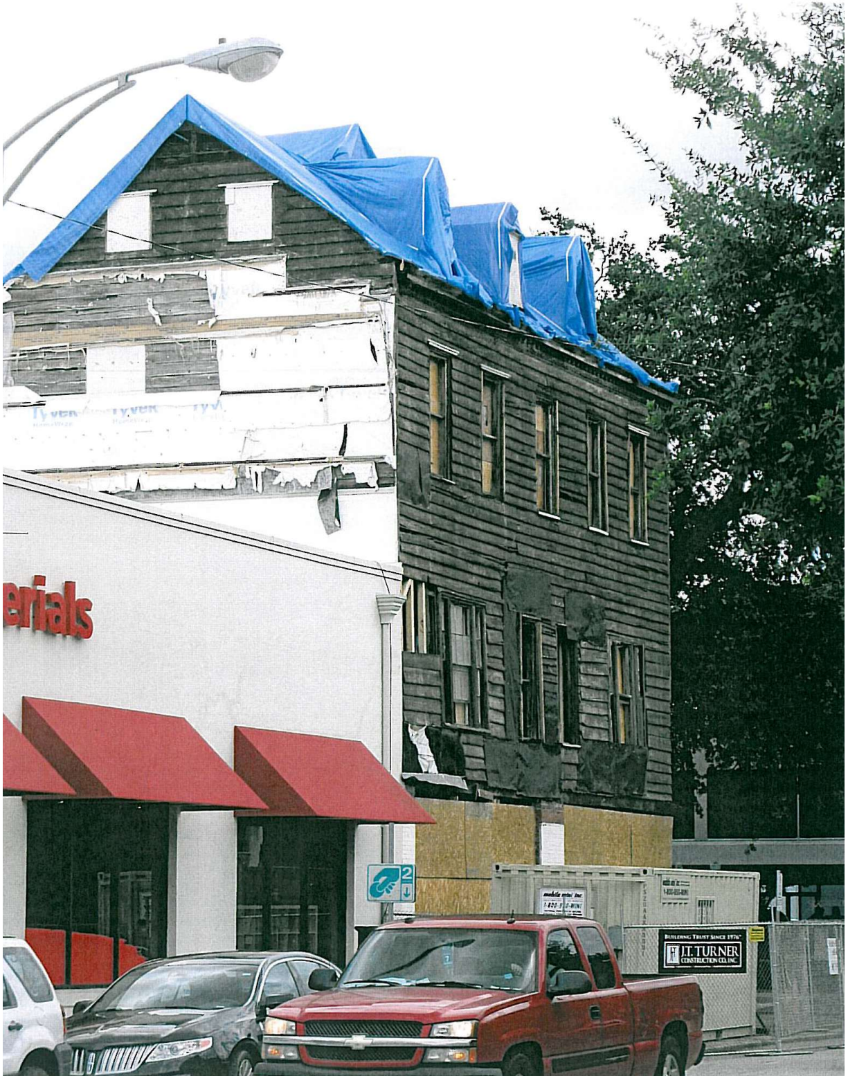
View of the west elevation before lowering of the building.
