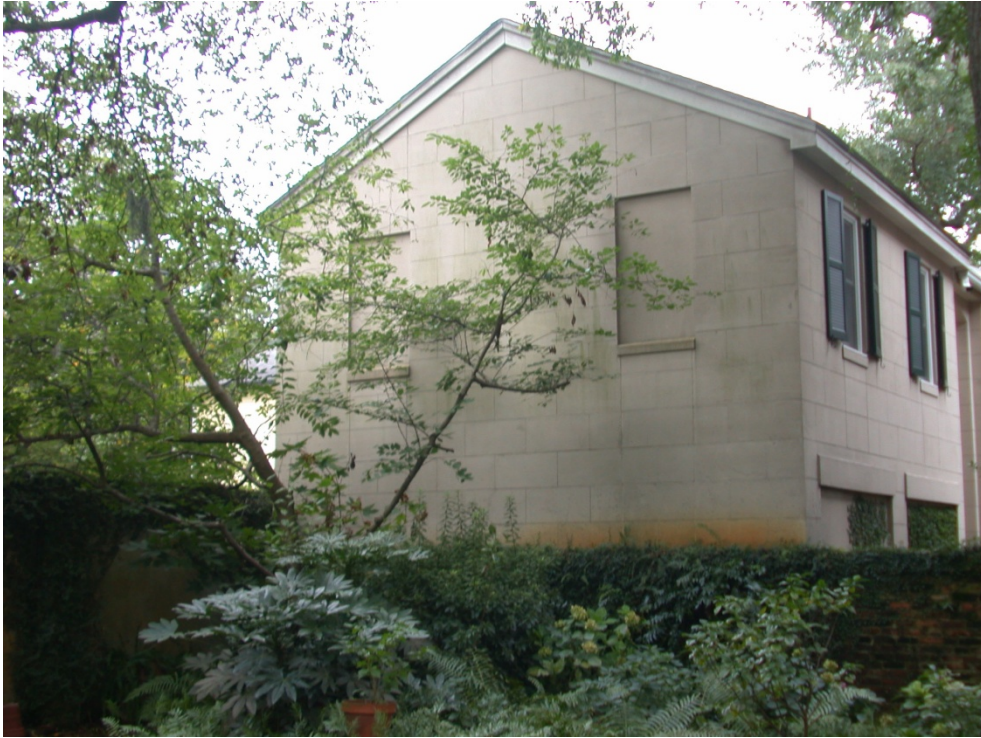
Existing Carriage House at rear of 220 East Hall Street (example of recessed stucco)
