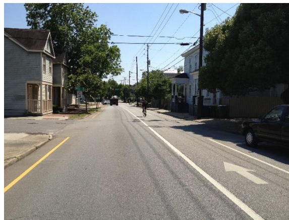
Price Street after May 2012: one regular travel lane, a bike lane, and on-street parking.
