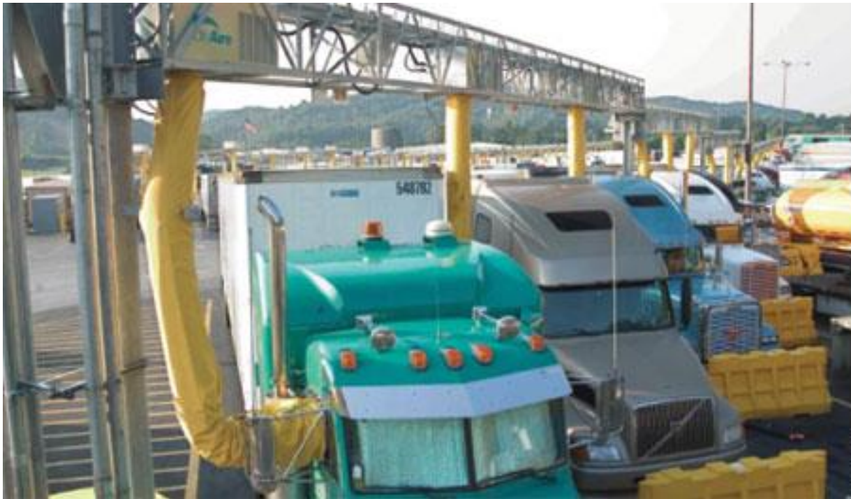
FIGURE 2.3 TRUCK STOP ELECTRIFICATION – KNOXVILLE, TN
