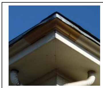
Repair: Pieced-In Wood Eave
