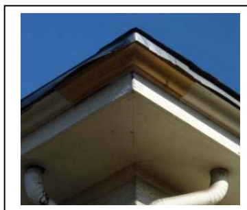
Repair: Pieced-In Wood Eave
