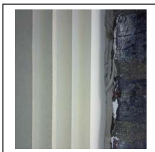
Routine Maintenance: Caulking and Painting
