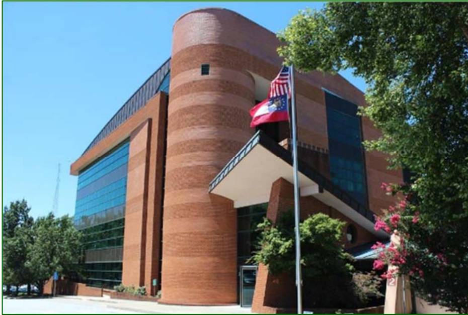
Figure 3-1: GDOT TMC in Atlanta
