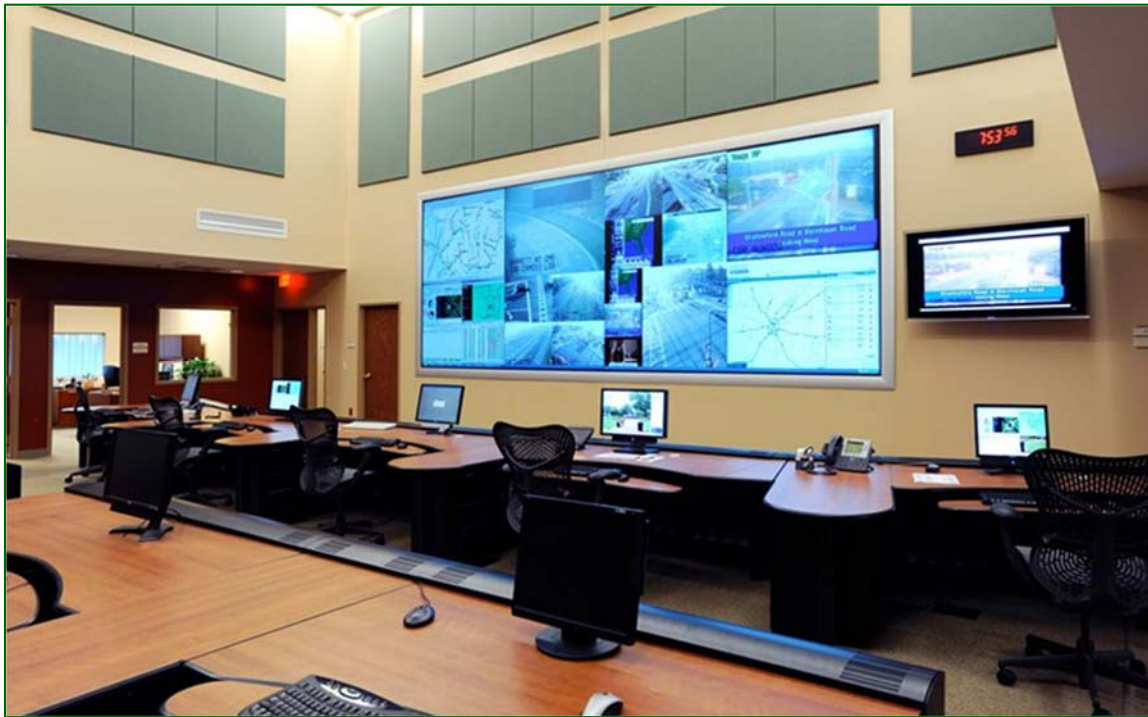
Figure 4-2: Cobb County RTMC Control Room
