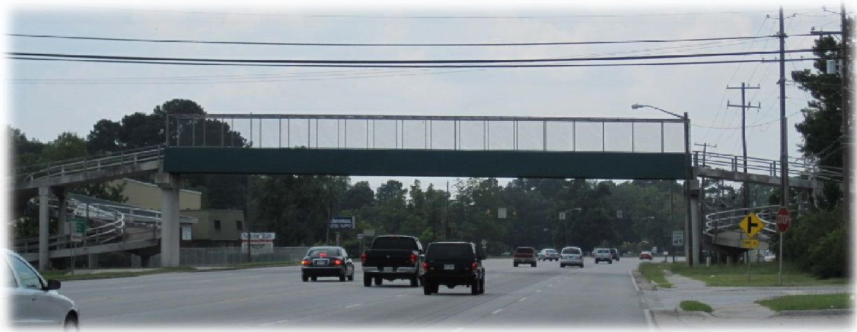
Figure 9 – Pedestrian Bridge over SR 21 in Garden City, looking north towards Rommel Avenue
