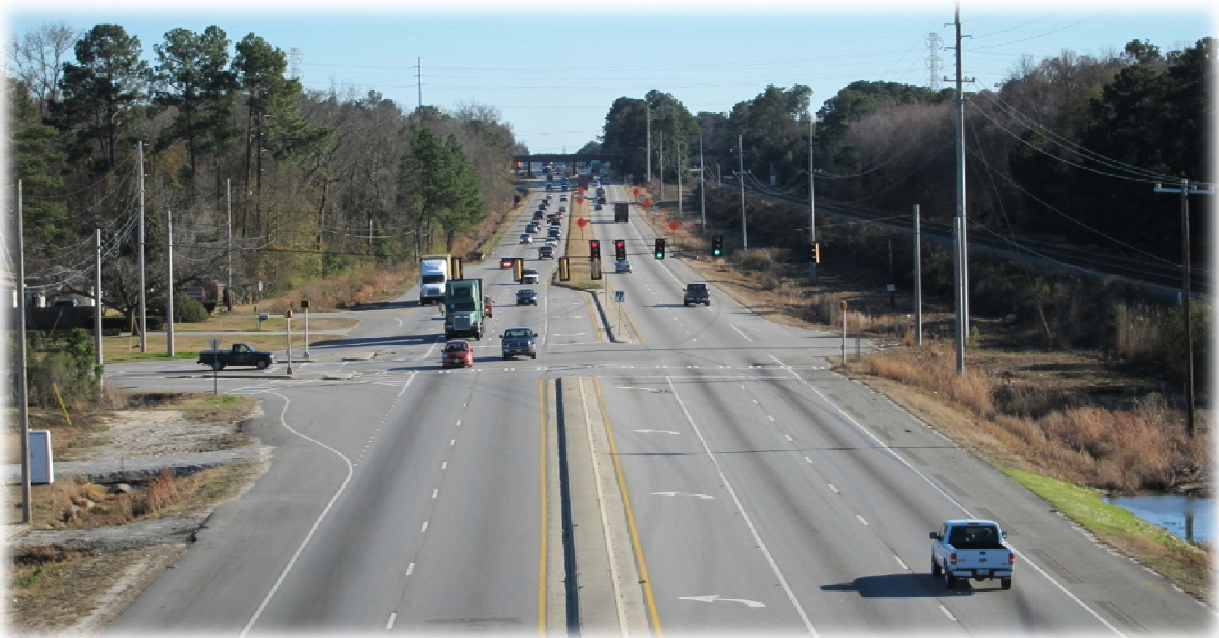
Figure 4 – Central Section – SR 21 as seen from JDL Parkway overpass looking south
