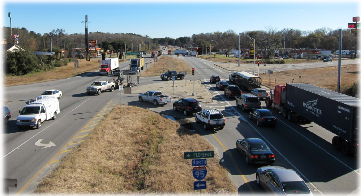
Figure 3 – Northern Section – SR 21 as seen from the I-95 overpass looking south
