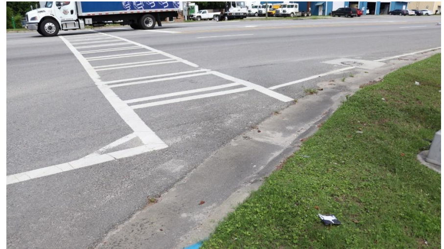
Image 4-20: Existing Multi-modal Infrastructure (Missing ADA Ramp at Intersection Crosswalk)
