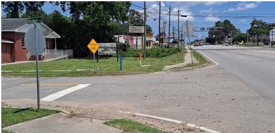
Image 4-17: ADA Ramps to Crosswalk at SR 21 and Bazemore Avenue
