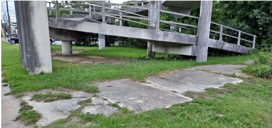
Image 4-16: Crumbling Path to Pedestrian Bridge on East Side of SR 21
