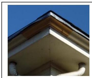
Repair: Pieced-In Wood Eave
