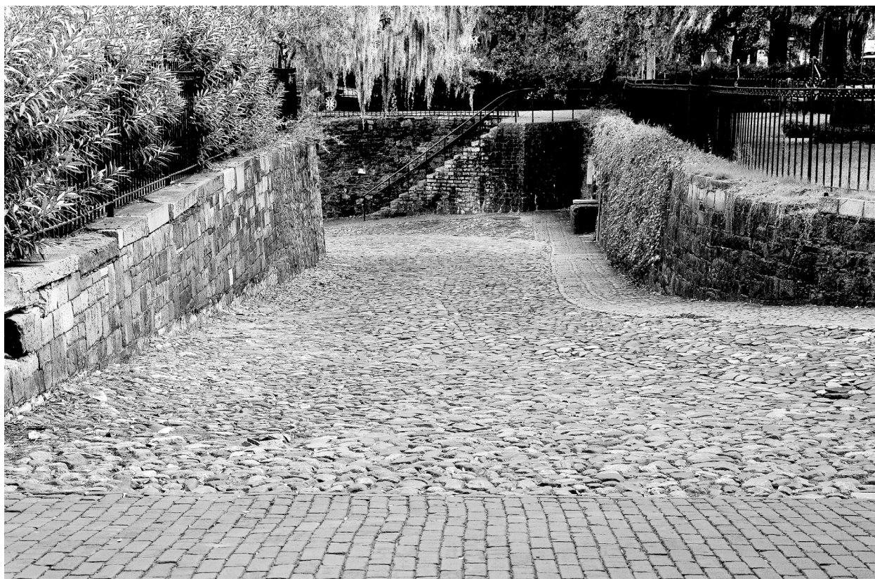
FIGURE 4 Cobblestone pavement on Lincoln Street Ramp, Savannah, 2011 (Photographs by author unless otherwise noted).
