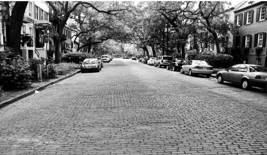
FIGURE 8 Red brick pavement on East Jones Street, Savannah, 2013, looking west from Drayton Street.
