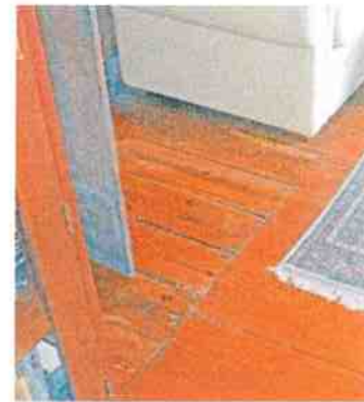
Figure 5. Break joint in floor boards in southeast front room.
