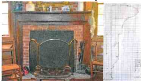
Figure 11. Left: Chimneypiece in north front room; Right: Section of the frieze and architrave. Note the quirked Greek ovolo and astragal molding.
