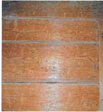
Figure 14. Beaded edge of sheathing boards, north front room.
