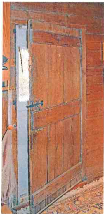
Figure 12. Batten door, south wall, south front room.
