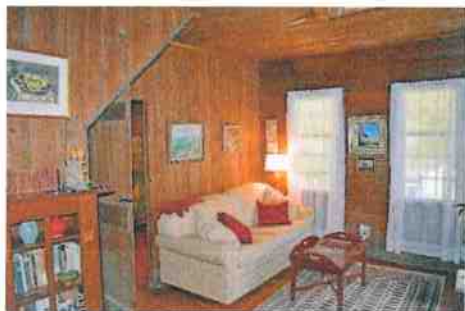
Figure 10. View of the south front room with vertical board partition separating it from the larger room. Note the board sheathing enclosing the staircase, the front wall, and the ceiling.
