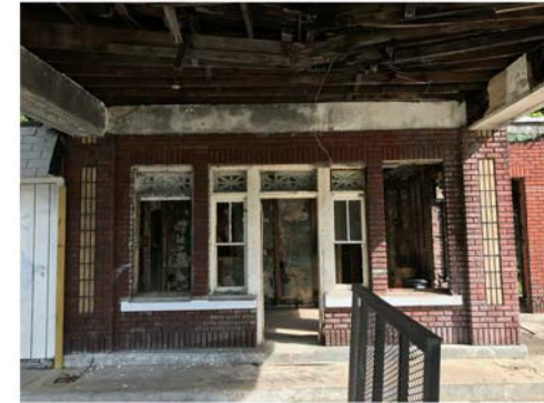
SOUTH FACADE - ENTRY
