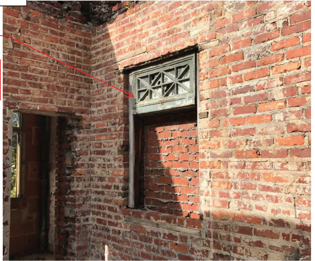
BRICKED UP WINDOW AT REAR
