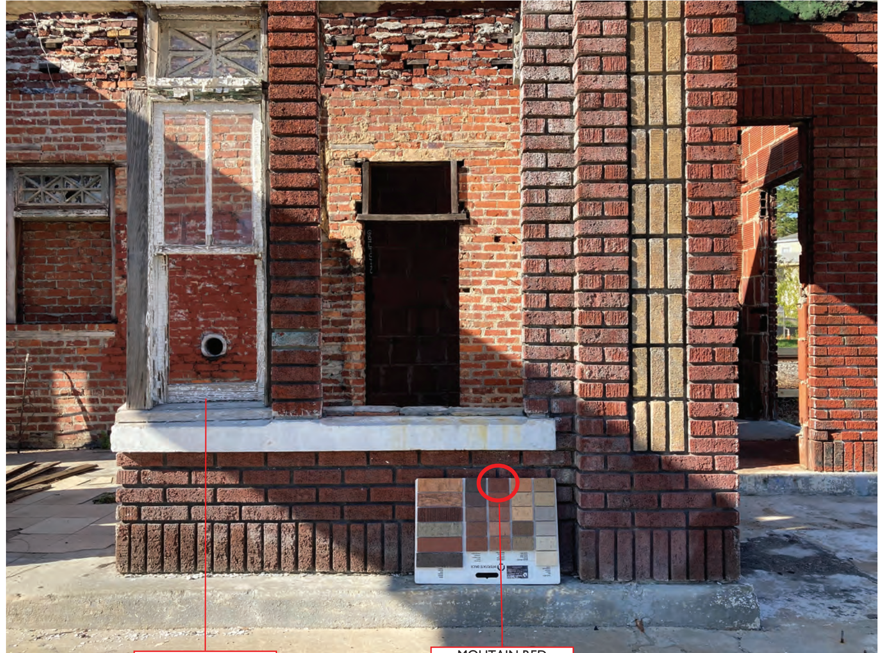
EXISTING WINDOWS - PAINTED WHITE
