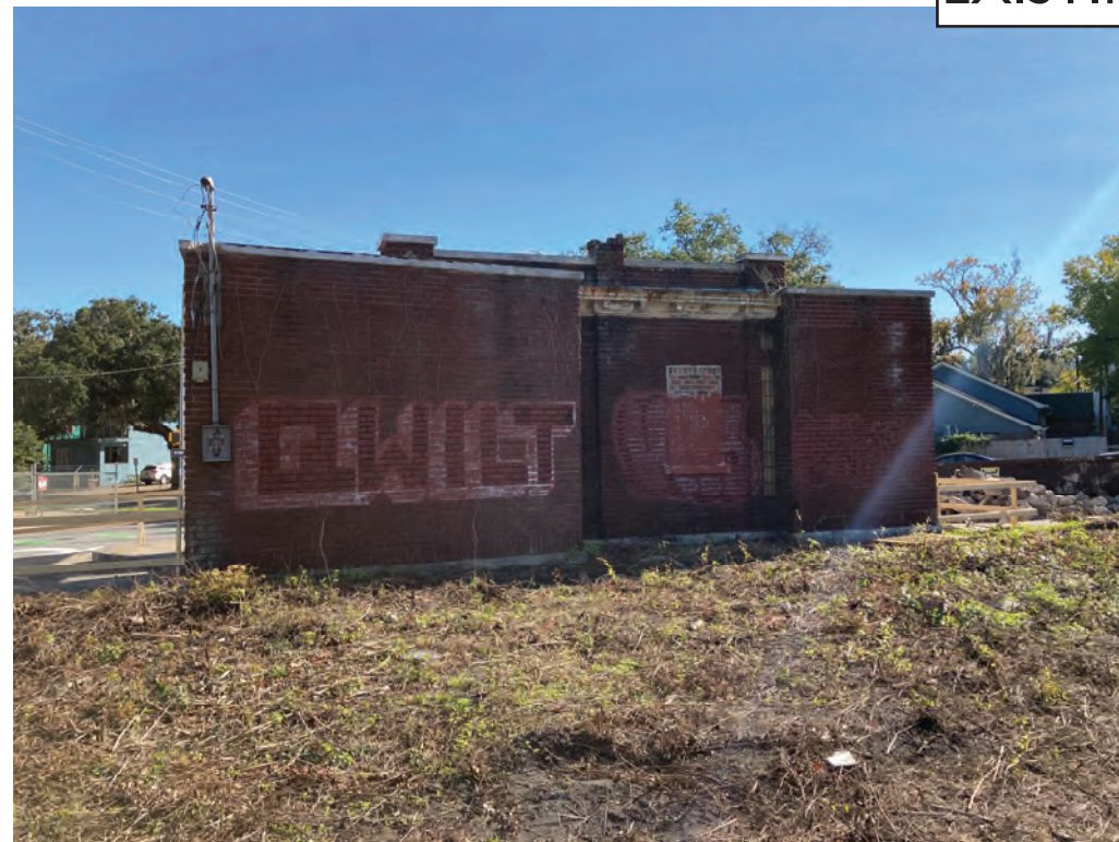
REAR ELEVATION - FACING RAILROAD TRACKS
