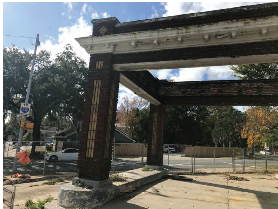
NORTH SIDE OF PORTE-COCHERE
