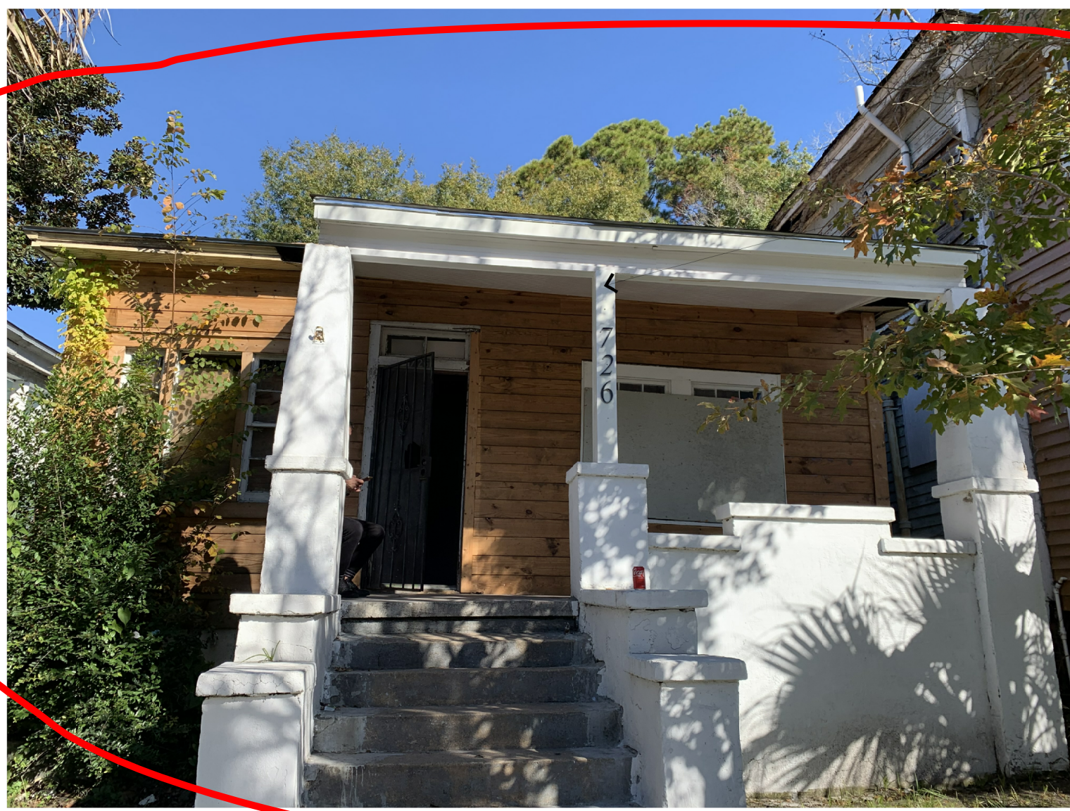
PHOTO OF AS-BUILT FRONT PORCH (4)
