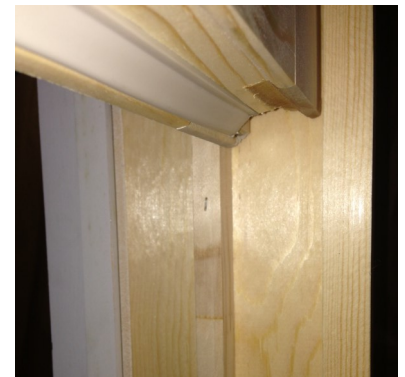
Side Jamb detail with Hidden Balance
