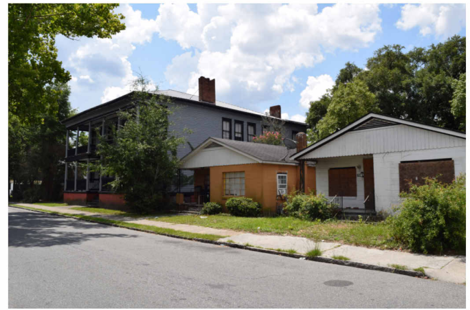
WEST 42ND ST. LOOKNG SE
