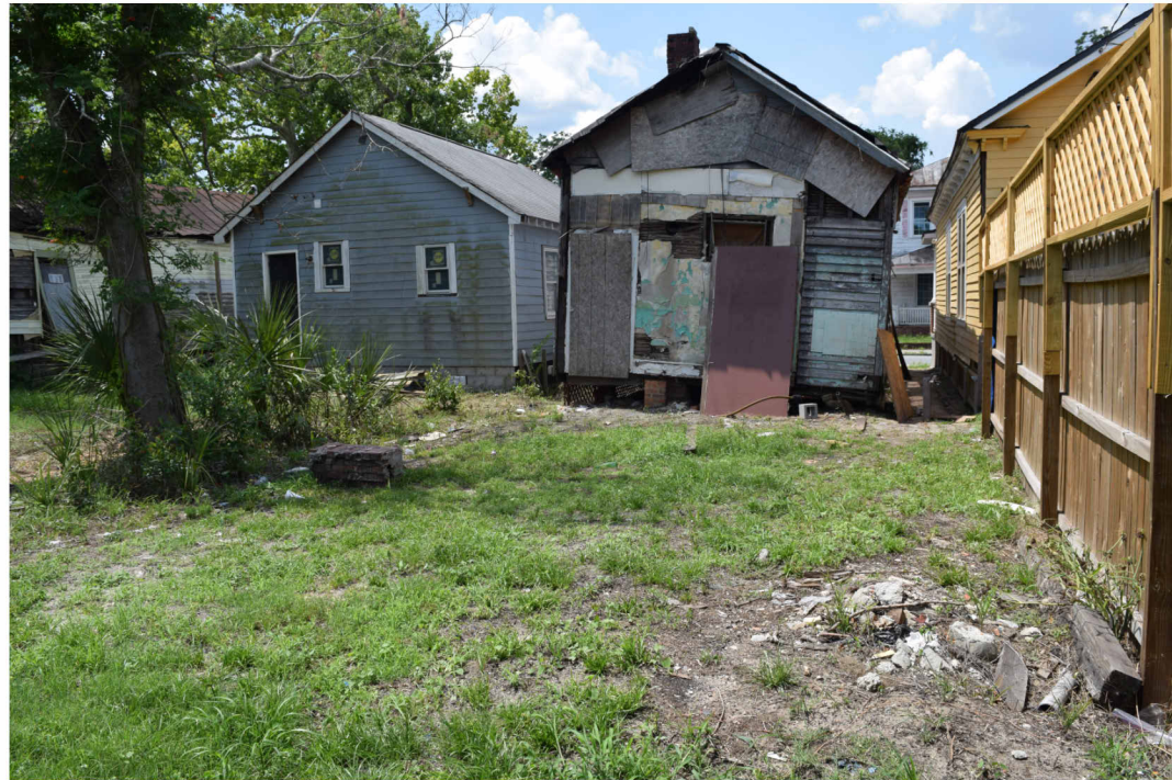
NORTH ELEVATION AND REAR YARD
