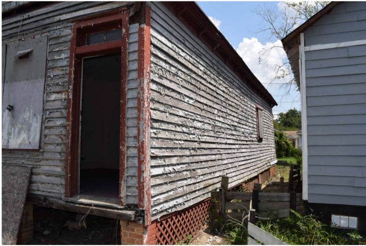
SOUTH AND EAST ELEVATIONS
