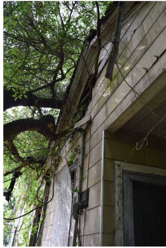
NORTH ELEVATION DETAIL
