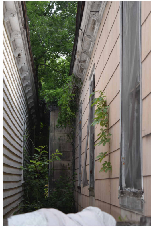
WEST ELEVATION - NORTH END
