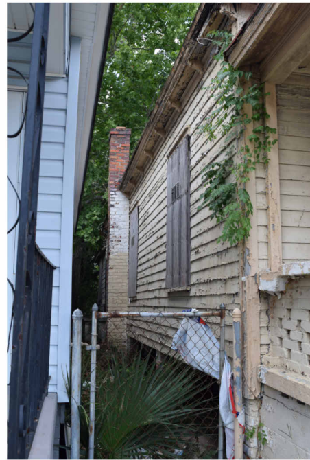
WEST ELEVATION - SOUTH END
