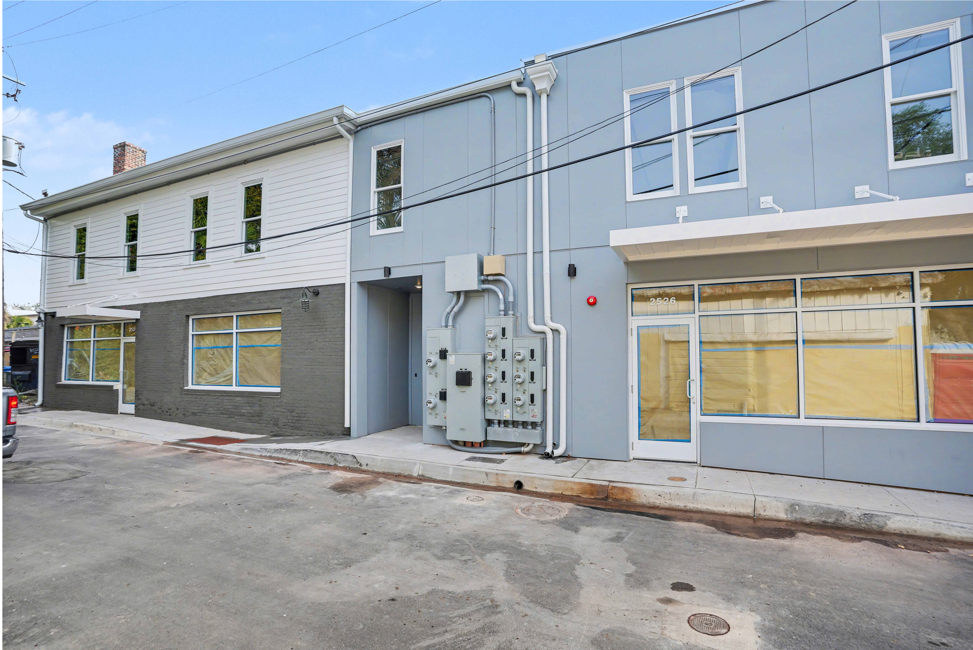
CURRENT PHOTO - WEST SIDE "A"
