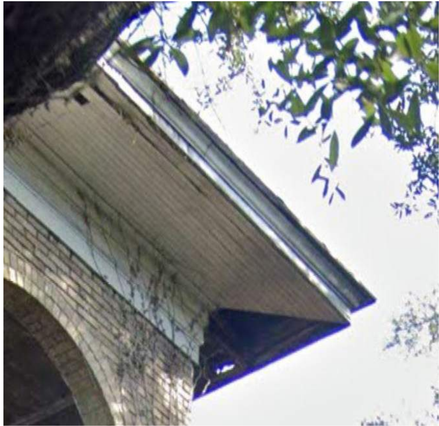
EXISTING CORNICE BEFORE IT WAS REMOVED
