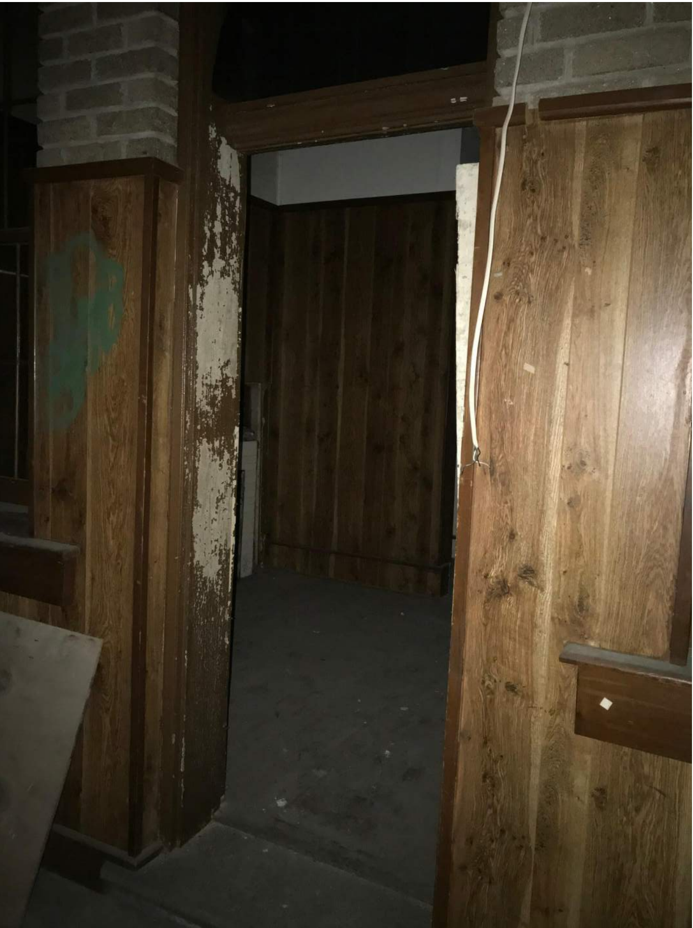
NOTE: SOME BALCONY DOORS HAVE BEEN REMOVED
