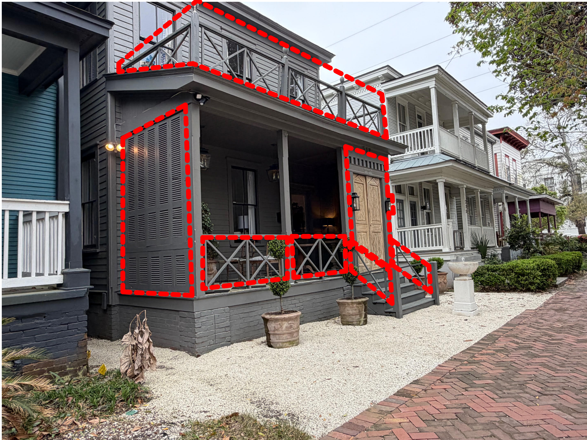
EXISTING PHOTO - LOOKING WEST
