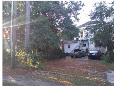
304 EAST 34TH STREET REAR ELEVATION
