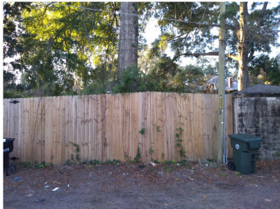
308 EAST 34TH STREET REAR ELEVATION
