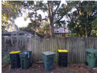
306 EAST 34TH STREET REAR ELEVATION
