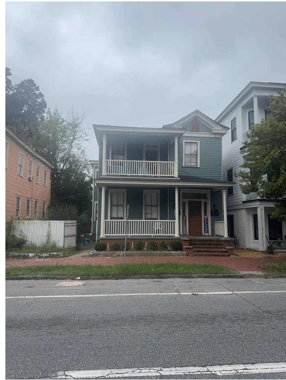
FRONT (FROM STREET)
