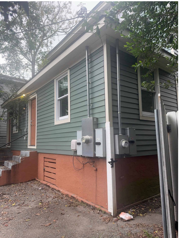
WEST (REAR CORNER)
