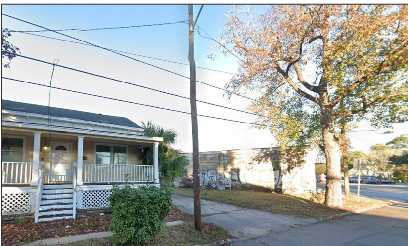
View from West 43 rd Street facing the rear elevation and showing the closest contributing building.
