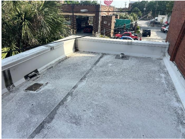
Lower Roof at Rear of Church
