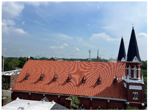
Roof (South Side)
