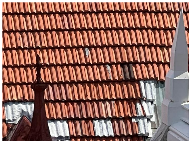
Missing tile, poor tile to metal pan termination
