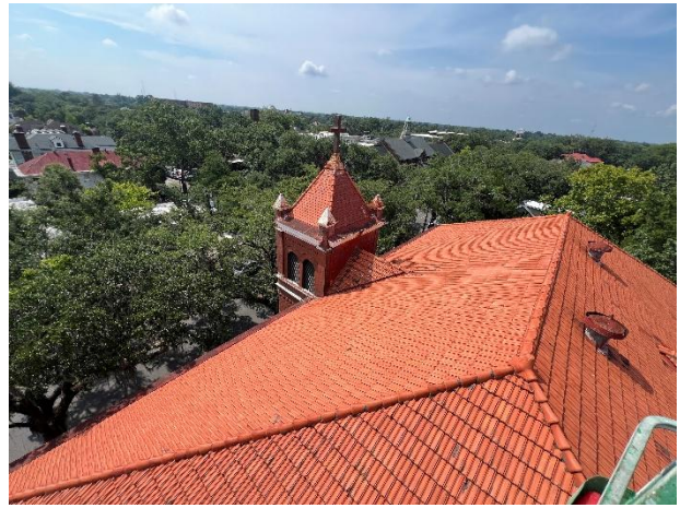
Overview of Roof
