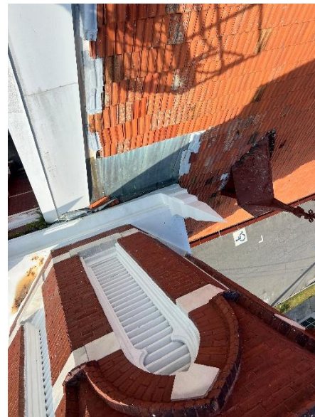
Missing tile, poor tile to metal pan termination
