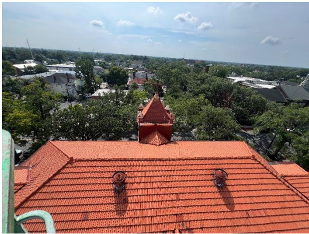
Overview of roof
