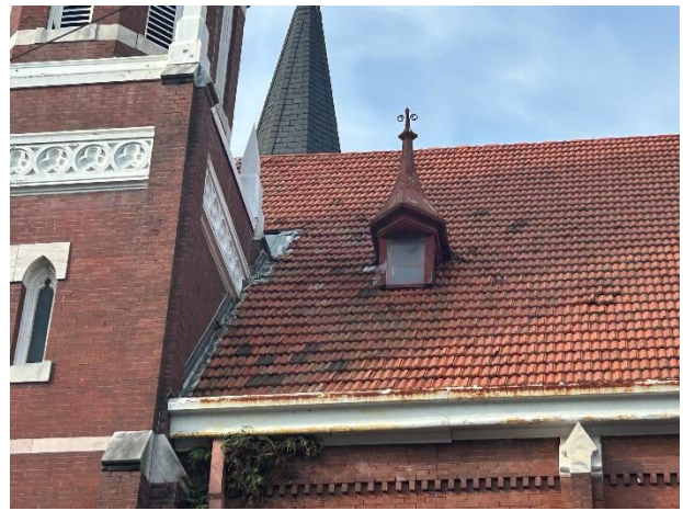
Dormer on North side of roof
