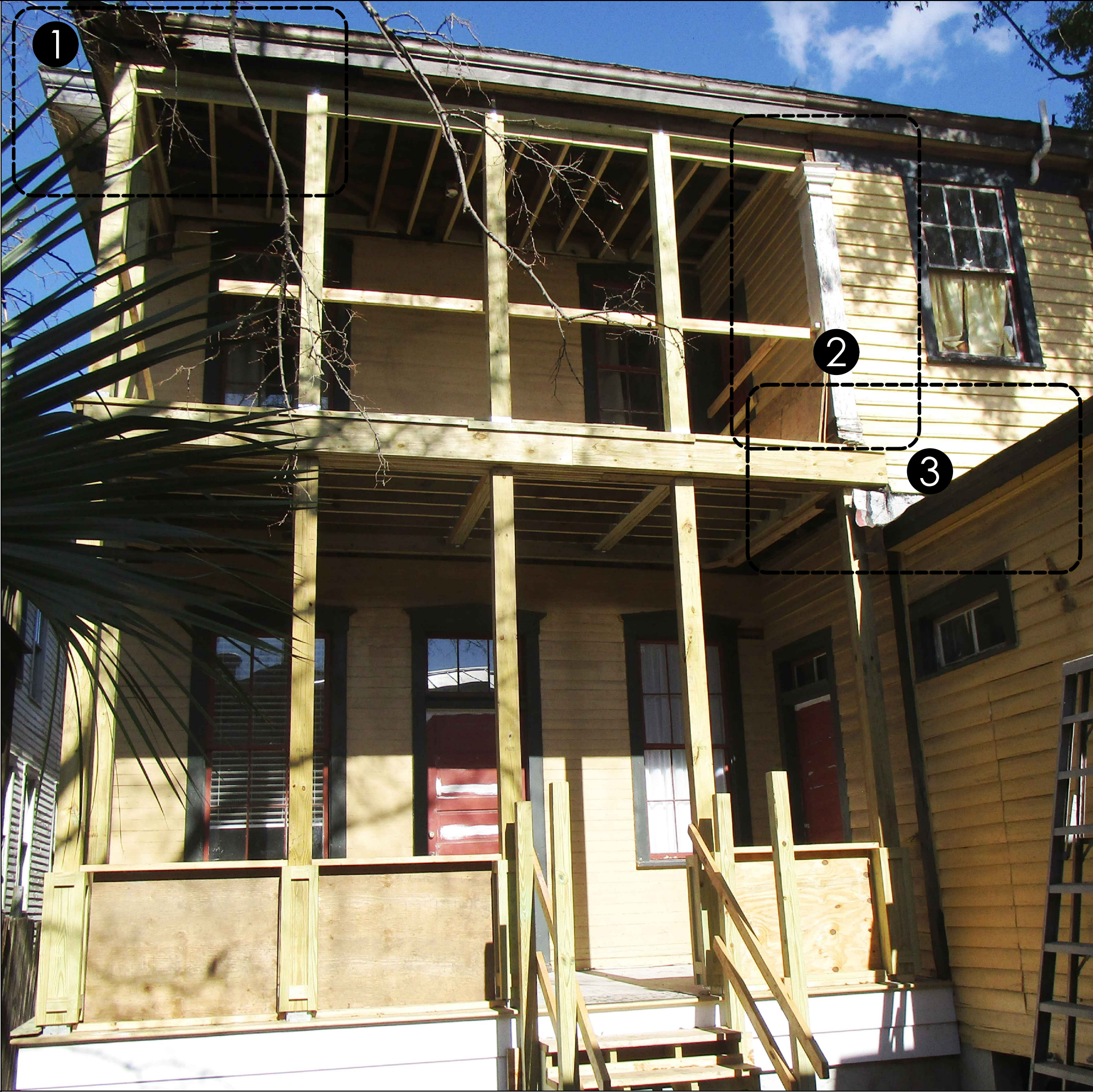
2 REAR PORCH (EXISTING)
