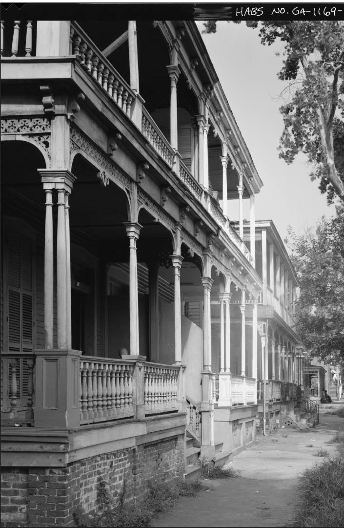
3 HABS PHOTO 1979: 209 & 211 W WALDBURG - FRONT PORCH
