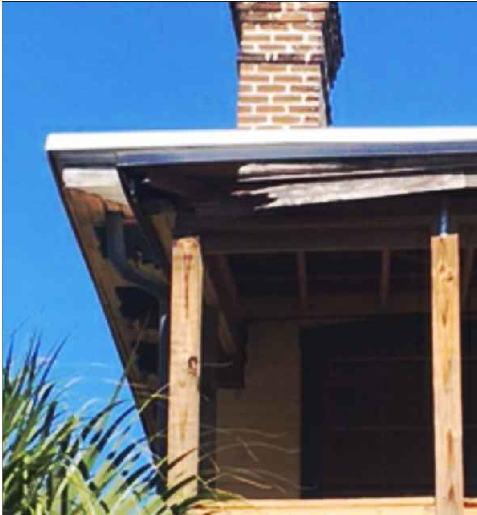
1 CORNICE & ARCHITRAVE AT SOUTHWEST CORNER
