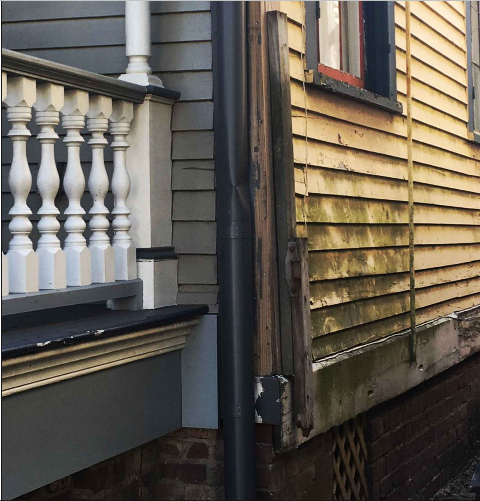
3 SHIPLAP SIDING AT WEST ELEVATION
