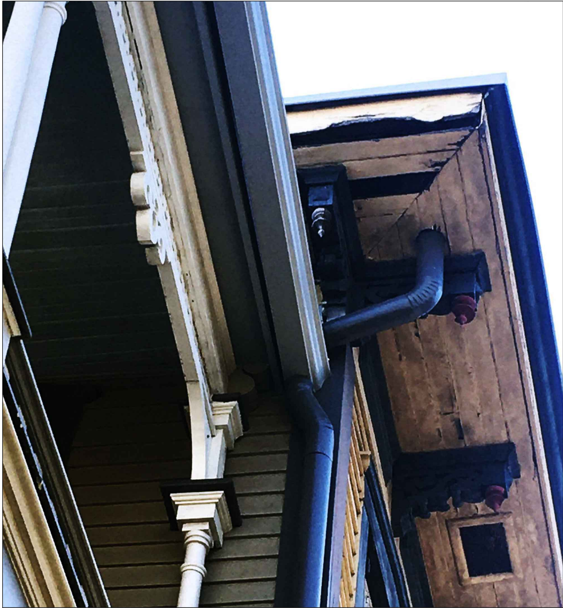
1 SOFFIT AND FASCIA AT NORTHWEST CORNER
