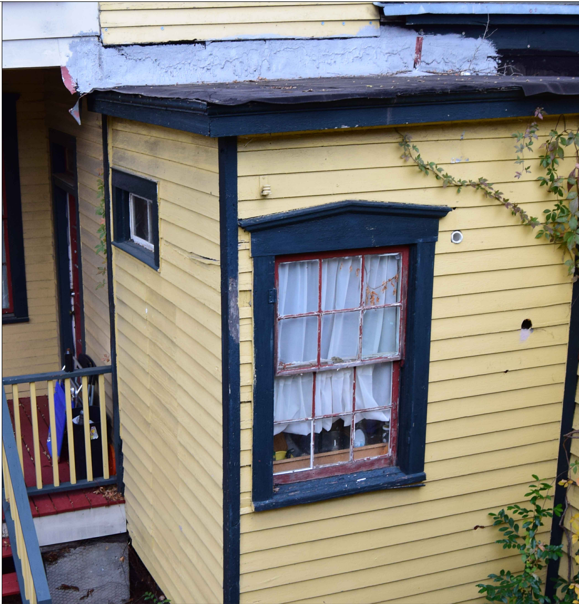
3 ROOFING AT SHED ROOF
