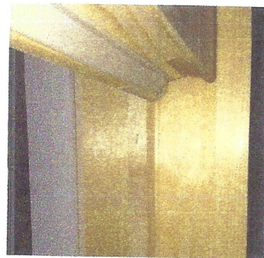
Side Jamb detail with Hidden Balance
