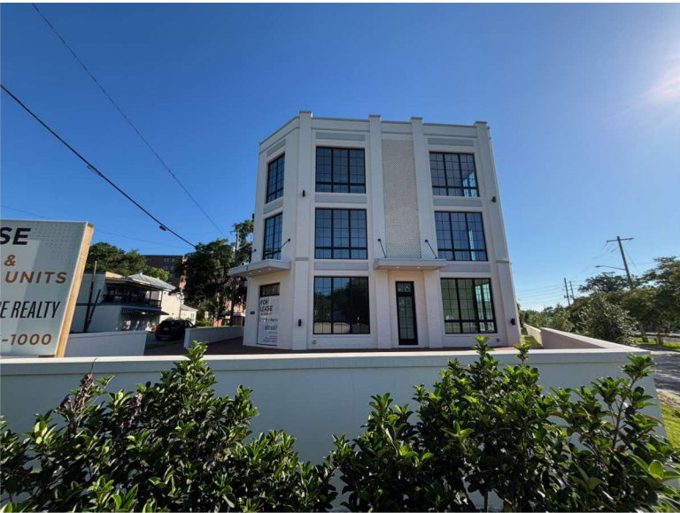
VIEW OF BUILDING FROM S
