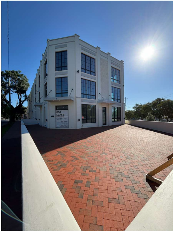
VIEW OF BUILDING FROM SW
