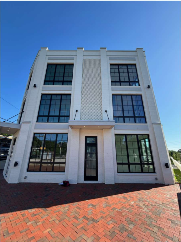
VIEW OF BUILDING FROM S W/IN PATIO SPACE
