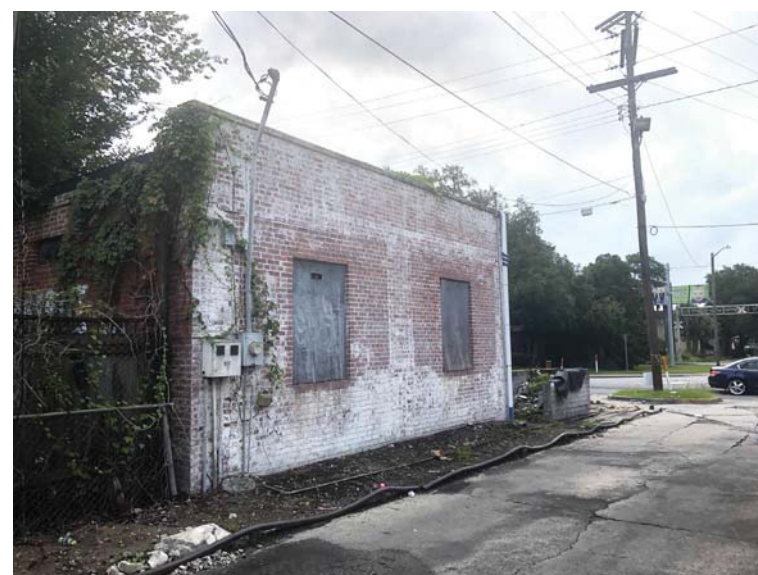
EXISTING SOUTH FACADE
