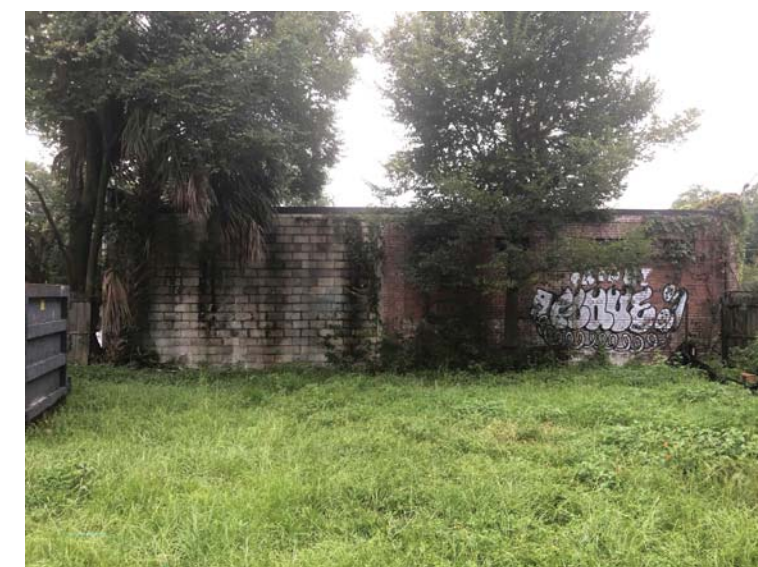
EXISTING WEST FACADE
