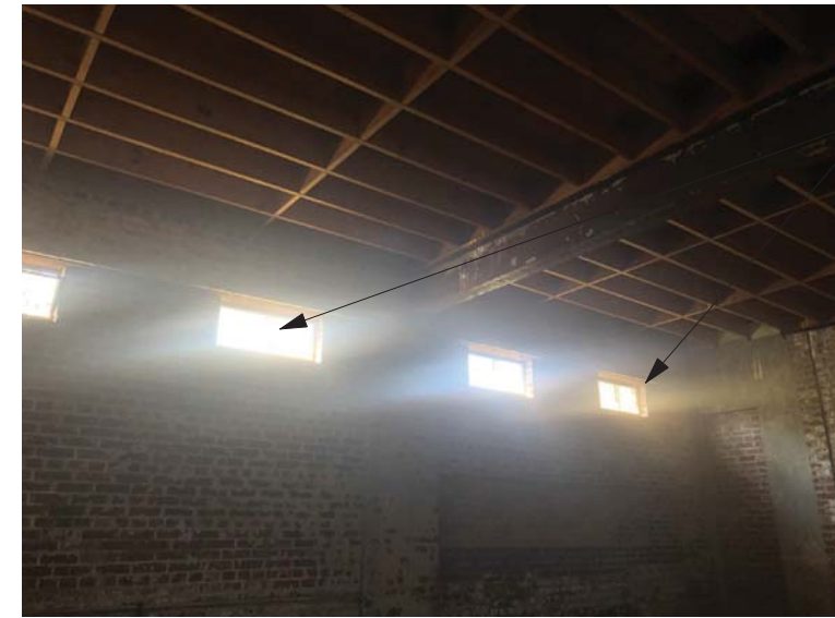
EXISTING, 2 LITE AWNING WINDOWS ON SOUTH WALL
