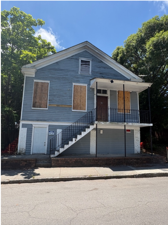
Façade (North Elevation)
