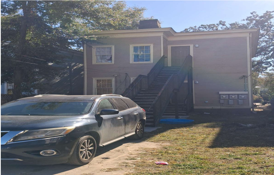
Photo 3: Adjacent property context — rear lane view showing neighboring structures.
