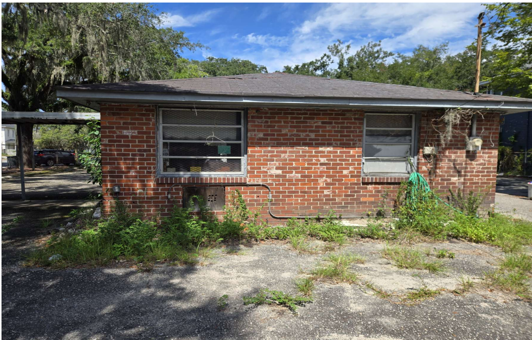
Photo 2: View of secondary brick structure on parcel — mid-century construction, aluminum windows, vacant and overgrown.
