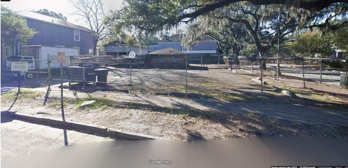
Photo 1: Current site conditions at 2300 MLK Jr. Blvd / future 415 W. 39th Street — site cleared and fenced (Google Maps, Nov 2025). Subject lot to be created via subdivision following demolition COA approval.
