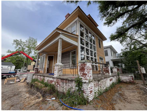
VIEW OF STUDIO FROM COURTYARD ENTRY
