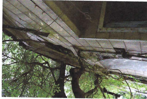
NORTH ELEVATION DETAIL
