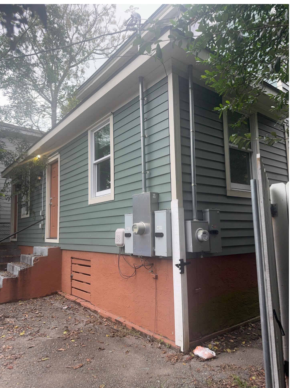
WEST (REAR CORNER)
