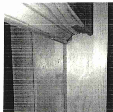
Side Jamb detail with Hidden Balance
