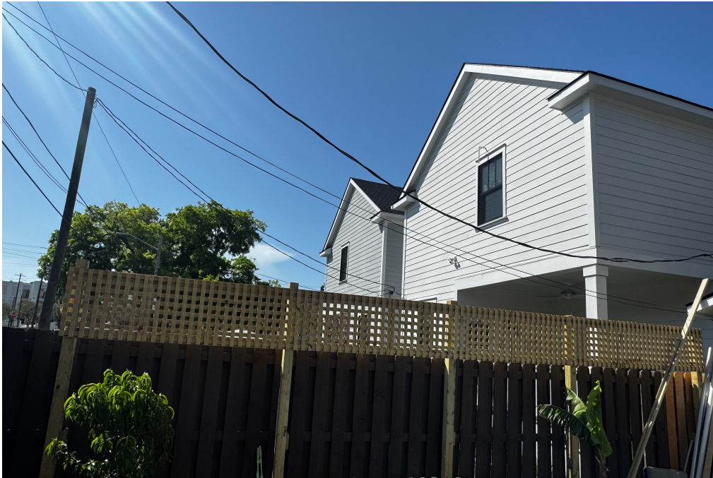
Lattice is 2 feet high in addition to the existing 6ft fence.
