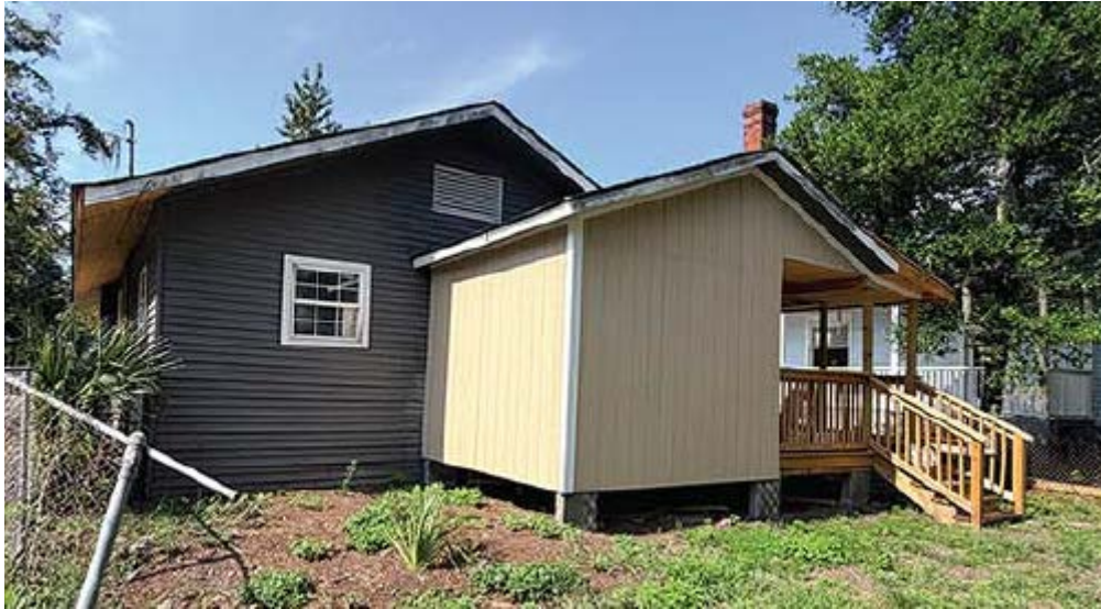
4. Current condition with the enclosed bathroom and new exterior porch and stairs
