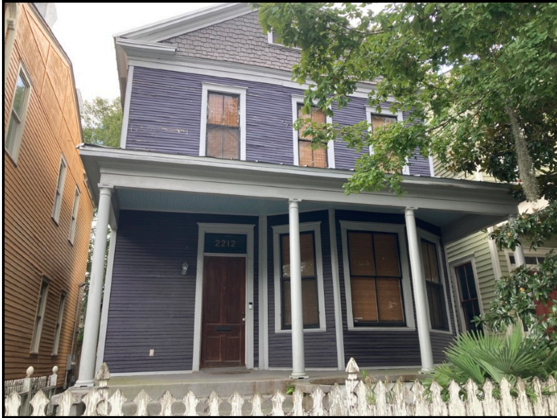
Front view of house on Barnard Street. Siding and trim in good condition. A few clapboards in the top section will be replaced if needed.
