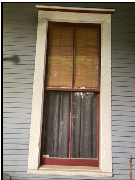
Window and trim in good condition. Not to be replaced.
