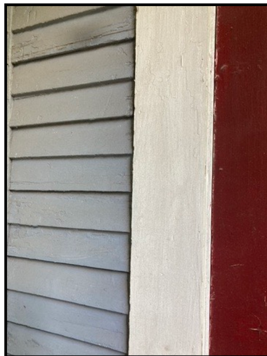
Close-up of original style siding and trim in good condition.
