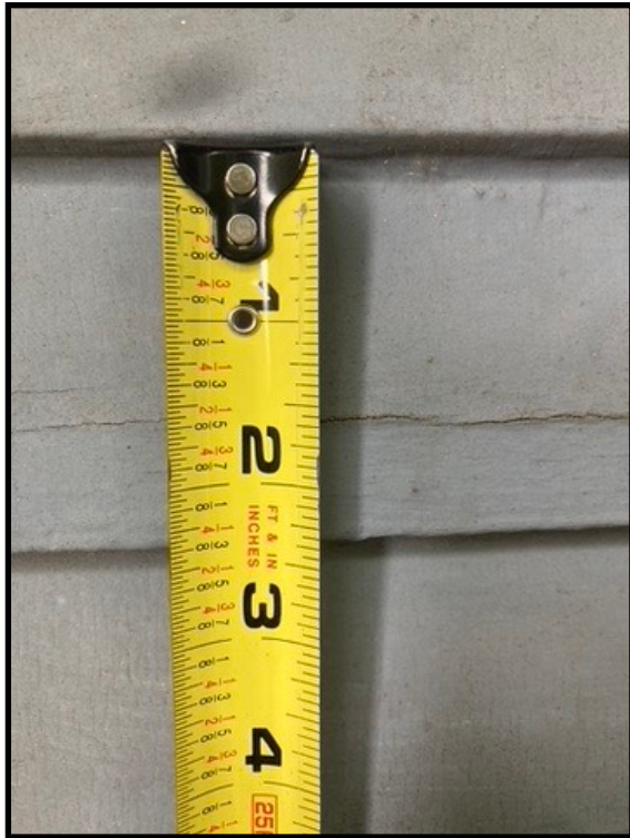
Close-up of original style siding showing profile and 3" reveal.
