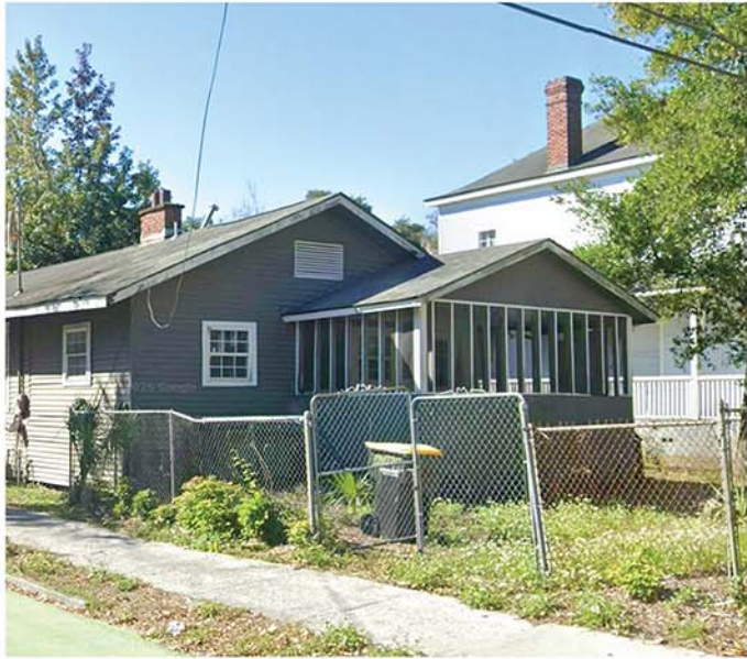
View of Rear Porch (Not Original to Cottage)
