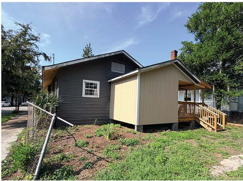
View of Rear Porch (Partial Enclosed) Work Completed without a COA
