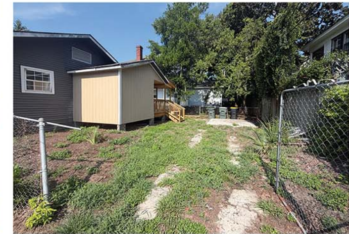
Photo 3: View from Lincoln Street
